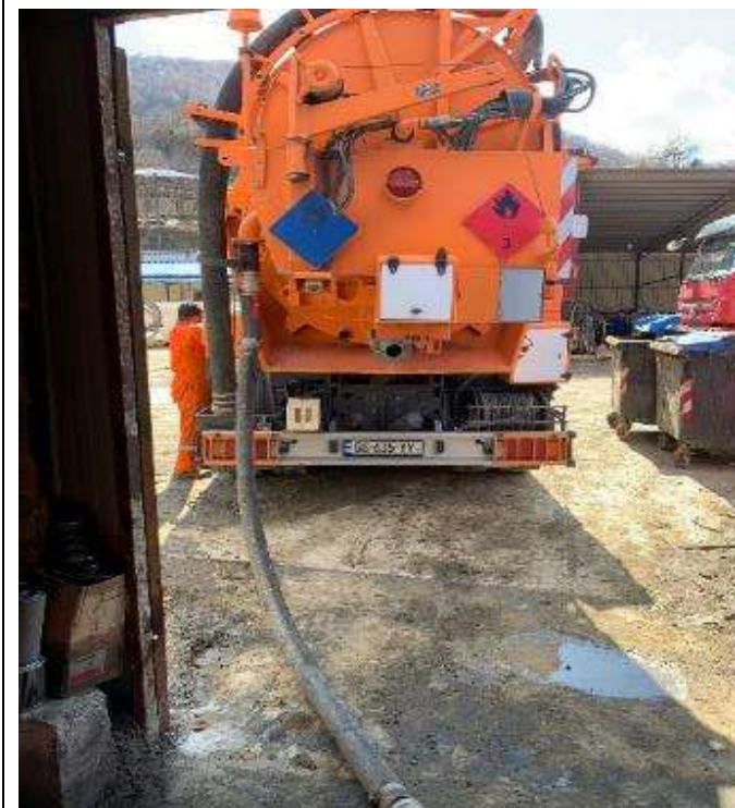
Waste Oil collection from the site by Subcontractor in March 2021
