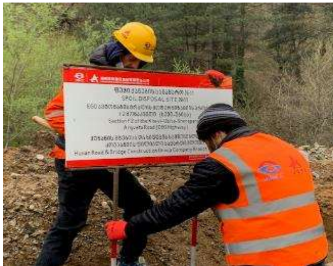
Information banners were installed at the spoil disposal sites #6,7,9,11 and 12.
