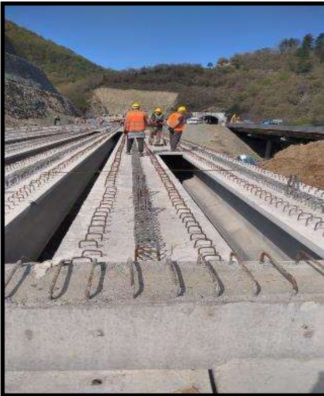
Guard rail required at Bridge# 5
